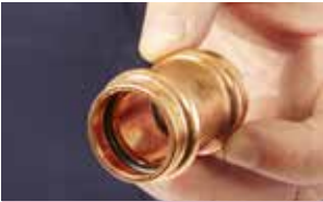
6. Ensure the O-ring is seated
