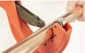
1. Cut the tube to length
