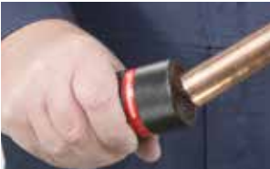
2. Deburr and remove all external sharp edges
