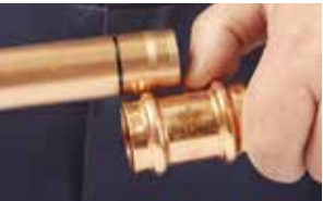
7b. Check the depth mark
